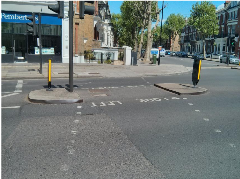
Photograph 2 – Example of islands - located on north-west arm of Shirland Road
